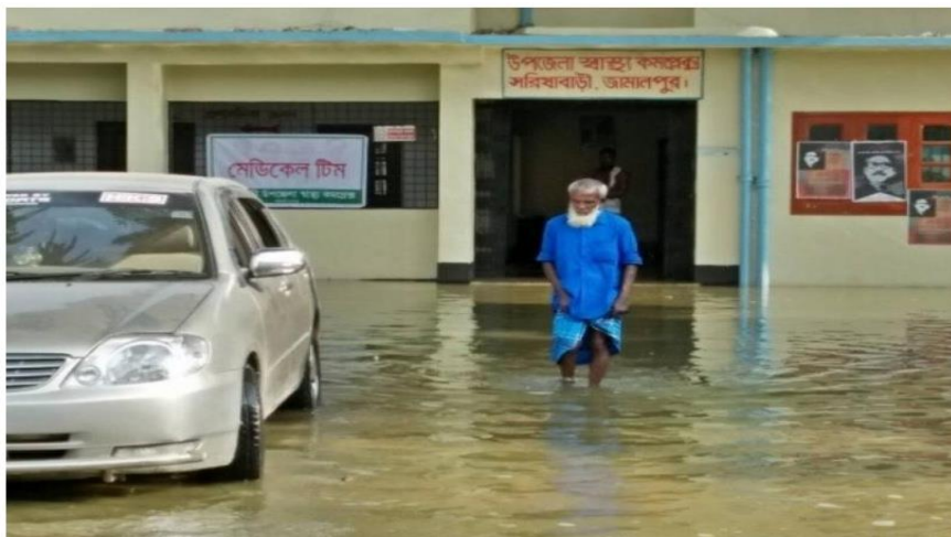
A flooded UHC in Dacope, Khulna
